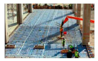
VaporBlock® is a high performance underslab vapor barrier designed to retard moisture migration through concrete slabs and concrete walls to protect your structure from:
